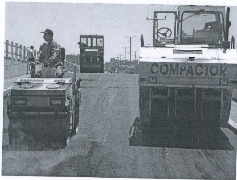
Asphalt Works (AL Zahra Box Culvert)
