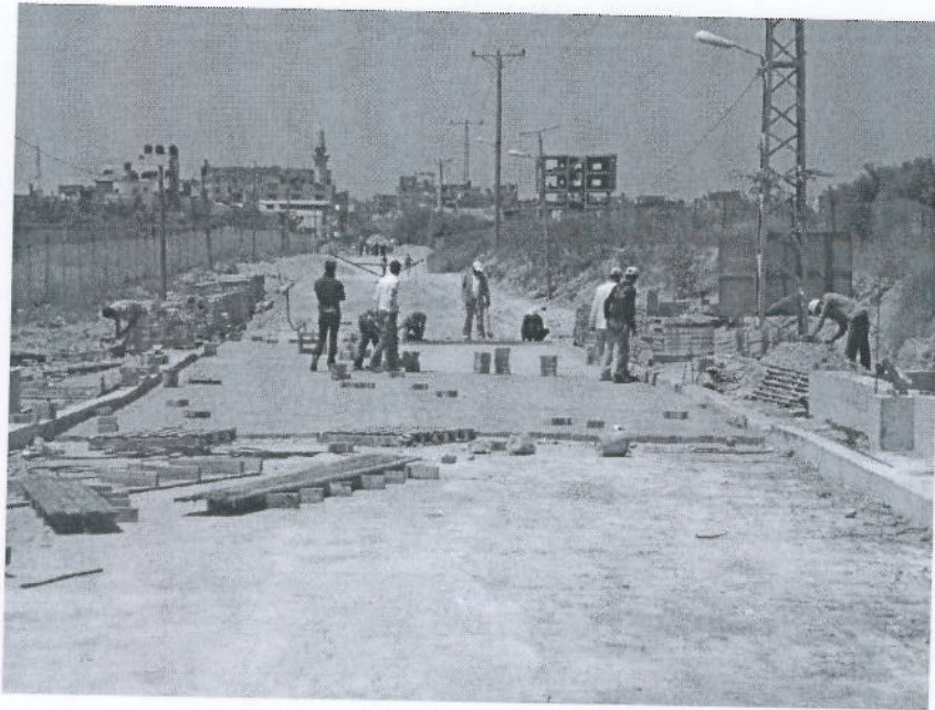
Interlock works (AL Zahra Box Culvert)
